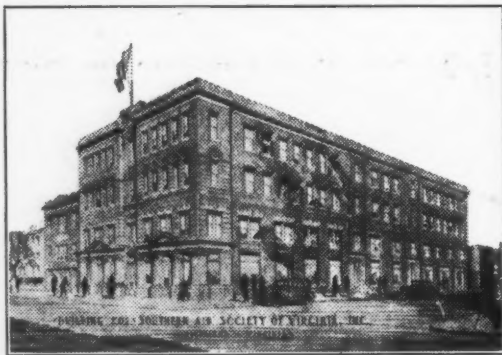
New Home Office Bldg. (Now under construction) N. W. Cor. Third & Clay Sts. Richmond, Va.
